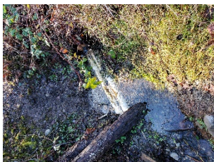
Erosion, invasive species & exposed pipes on creek bank at north east corner of park
